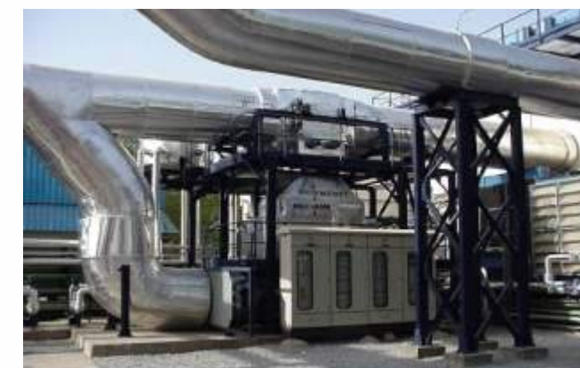
Waste Heat Recovery for Water tube type for Engine exhaust
