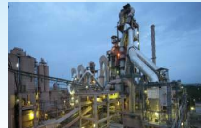
Waste Heat Recovery for Cement Plants
