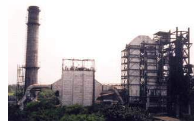
Waste Heat Recovery for Sponge Iron plant after ABC
